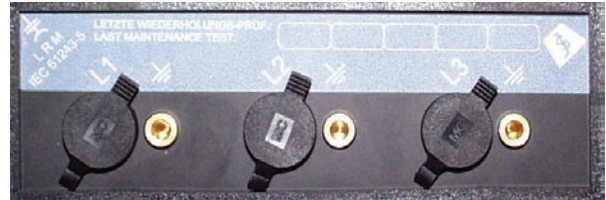
Fig. 6.9.1: Three phase LRM system
