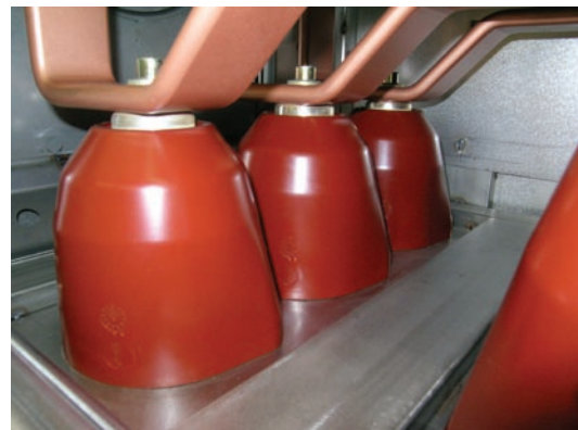
Fig. 6.8.1: View into the circuit-breaker compartment: test sockets
