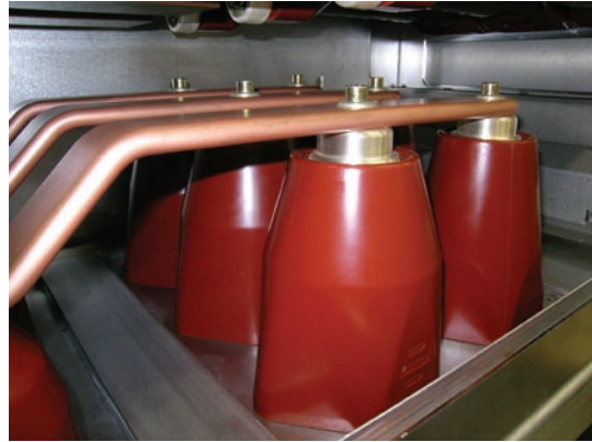
Fig. 6.5.1: View into the gas-insulated circuit-breaker compartment with inner cone sockets
